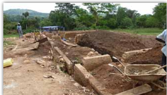
New classroom building for grade 2 and 3
